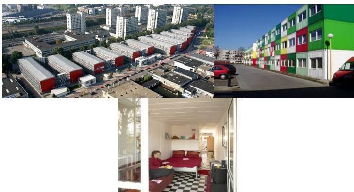
Figure 5: Kitwonen in the Netherlands is the largest container city in the world
